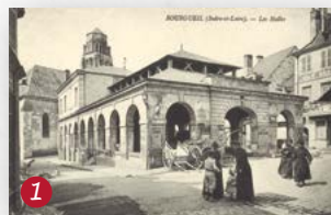
Les Halles: centre de la vie économique "Les Halles" (Market Halls): Centre of daily economic life
